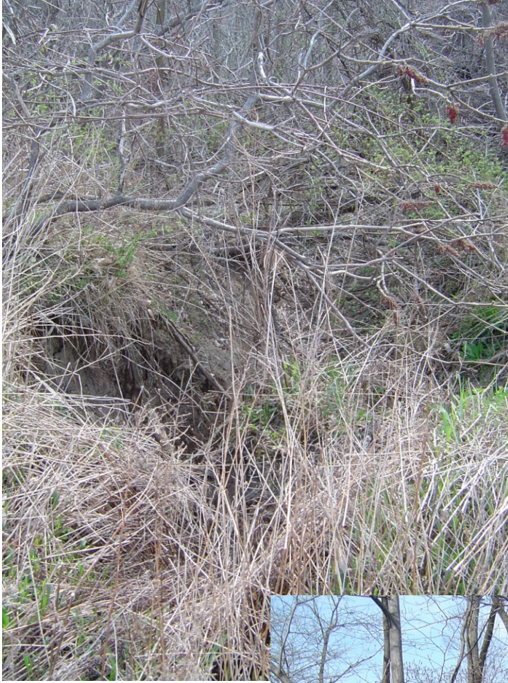
Photo 11: Shallow gully forming on slope of table lands west of Havens Lake Road (typical).
