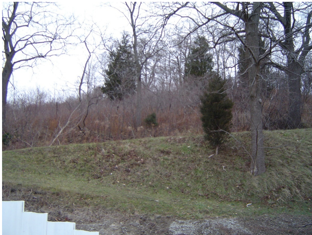
Photo 3: Slope near east end of marina parking lot.
