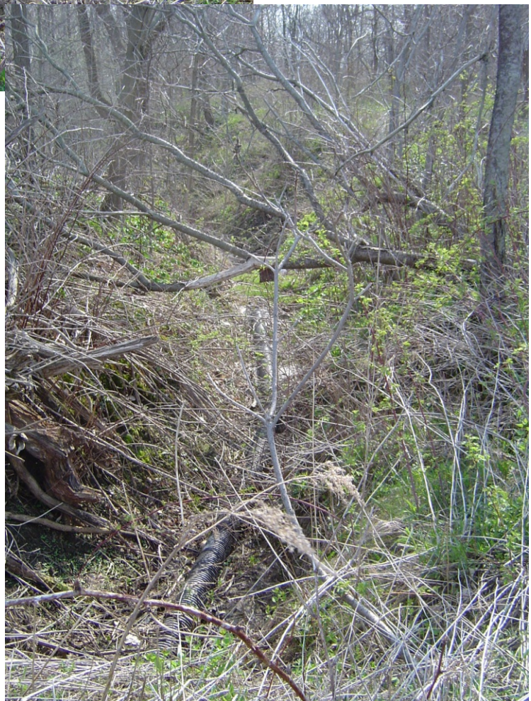
Photo 14: Drain pipe at top of gully forming south of Gray Line.
