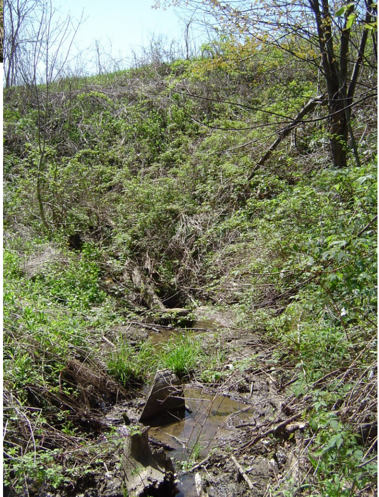
Photo 8: Culvert pipe at filled portion of gully east of Havens Lake Road and south of Gray Line, looking south.
