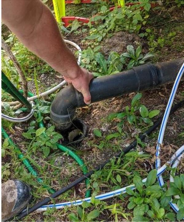
Figure 2.5 – Example Service Connection
