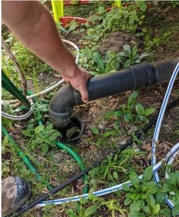
Figure 2.5 – Example Service Connection
